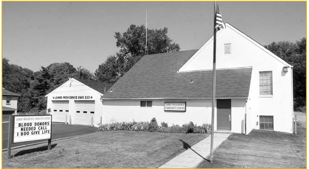
The Lower Providence Community Center on Hillside Avenue.
