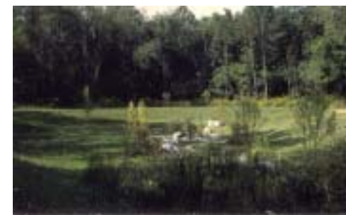
A basin with a naturalized low flow channel and additional landscaping.
