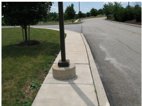
Incorrect light pole placement limits ADA accessibility.
