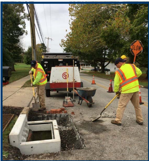
This inlet on Level Road was one of 53 that were reconstructed in during the year.
