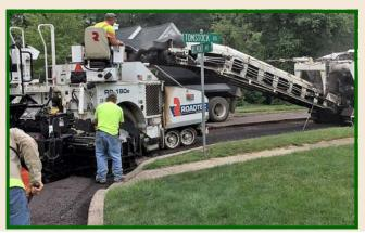
Cold in-place recycling work on Tomstock Road – the existing asphalt is being removed and reused.
