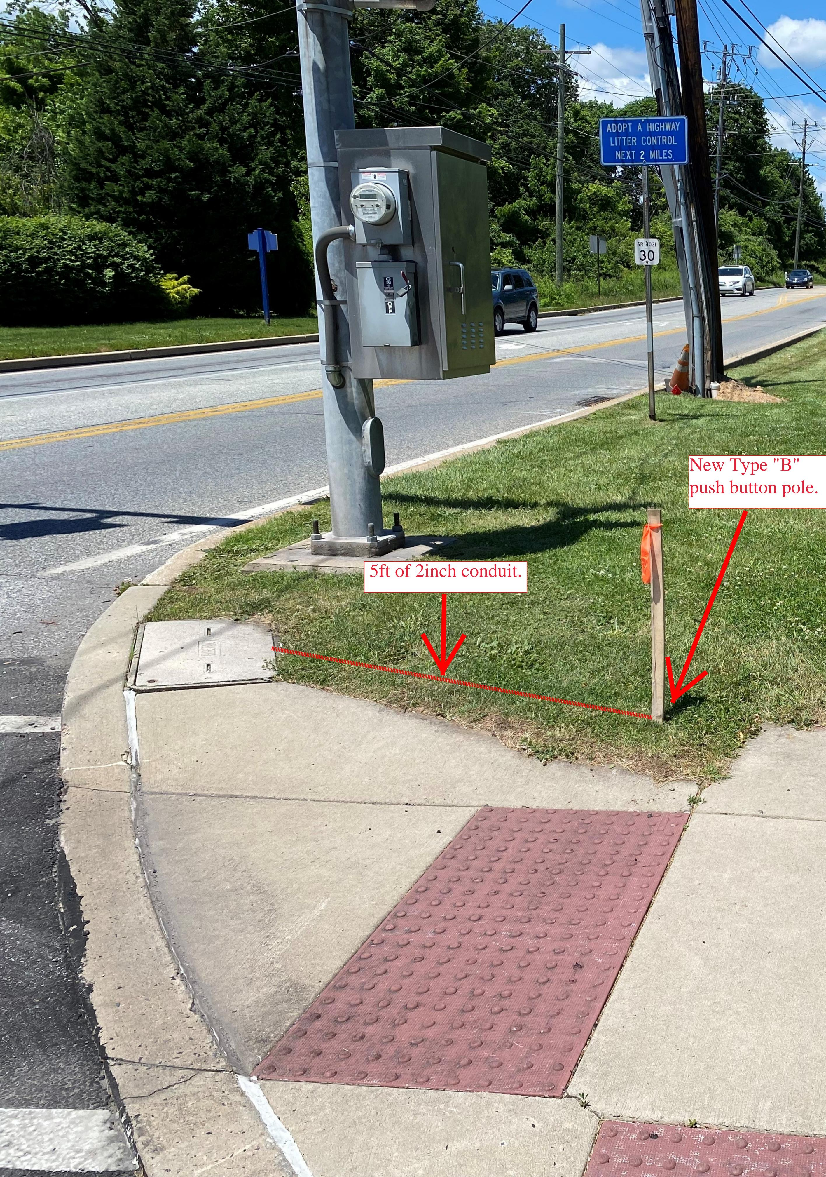
Replace existing Type "B" push button pole (wobbly) with new Type "B"pole & foundation.
