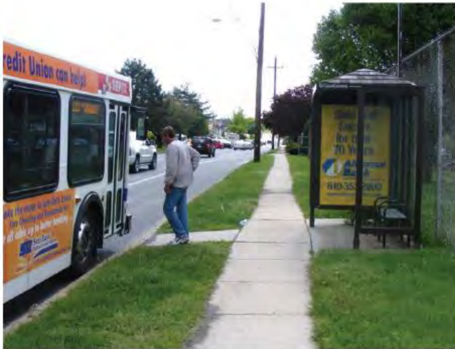
Passenger boarding bus from front door loading pad (Source: Delaware County Planning Department 2010)
